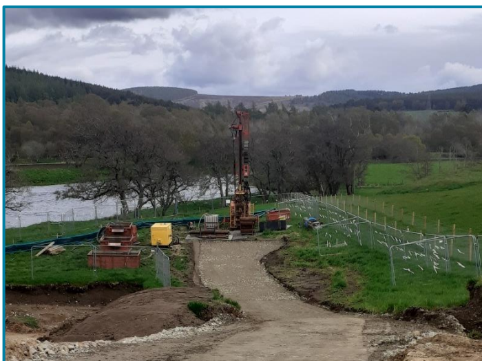
Figure 19: Drilling of a groundwater abstraction borehole at The Cairn
