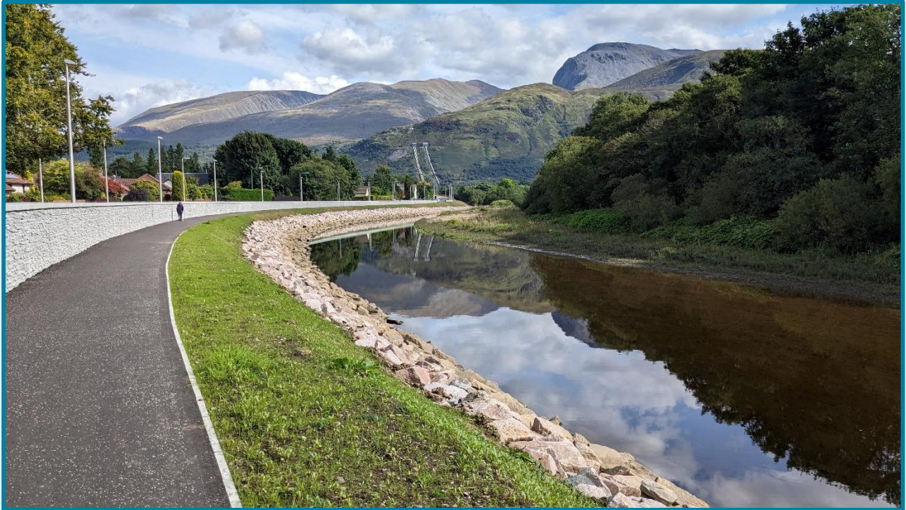
Figure 14: The River Lochy, Embankment and Flood Wall
