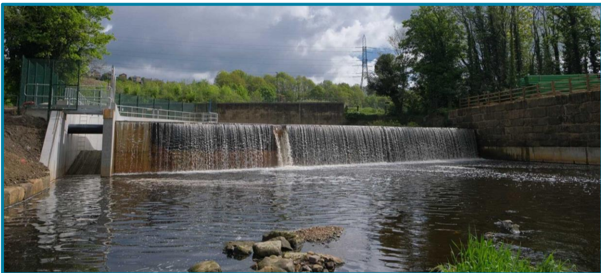
Figure 8: Niagara Weir stabilisation and fish pass on the River Don
