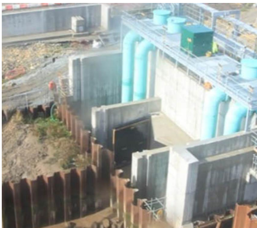
Figure 6: East Hull Pumping Station
